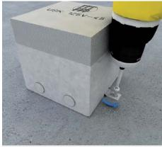
**1 | Floor box** Align floor box in dead centre as delivered. Bend open ears and fix to raw ceiling.
